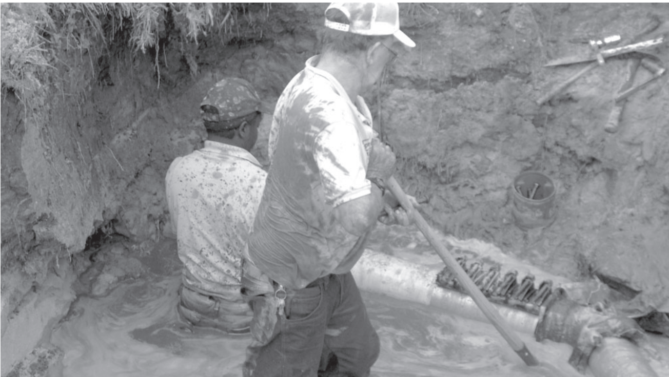
Pictured here are: Greg Gretz, right, and J.R. Clarke, left, doing what it takes to fix a water main break.
