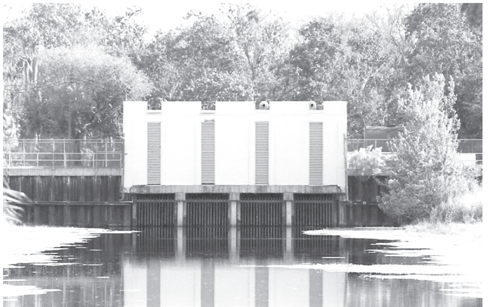
Outside pump station
