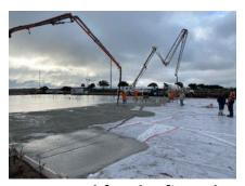
75 loads of concrete were used for the first phase of garages, and the steel frames are being installed
