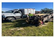
8" sewer force main being bored on Cozumel for phase two of Apex
