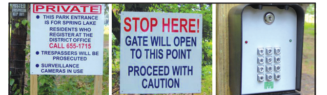
A new coded gate and surveillance system has been installed at the main entrance to the park, as well as the boat ramp. You can secure access by contacting the District Office at 655-1715
