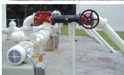
The recent shut down of the water plant was needed to install these new pipes and shut off valves to ensure quality water supply and service to our Spring Lake residents.
