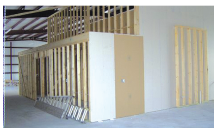
Work on the interior has begun, and plans are to move in by the end of July. This much needed complex will serve Spring Lake for many years.
