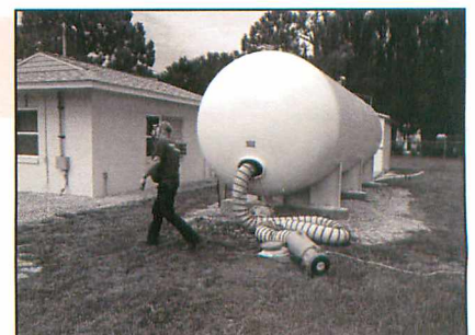
Water Plant Tank Inspection
