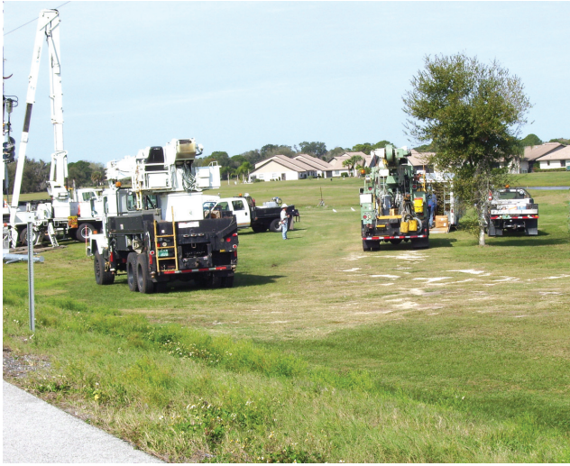
Progress Energy changing poles and wires in the District
