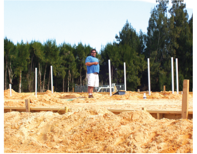
Plumbers working on the new maintenance facility
