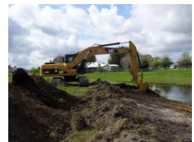
De-Silting Canals
