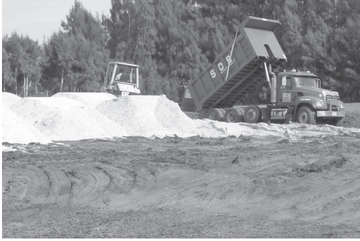
Close to 40 loads of sand were brought to the site for a solid foundation.
