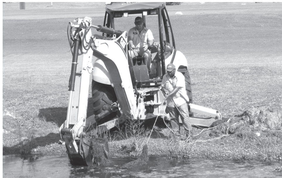
Foreman Randy Nelson operates the backhoe and Assistant Foreman Corey Jones extracts the hydrilla.
