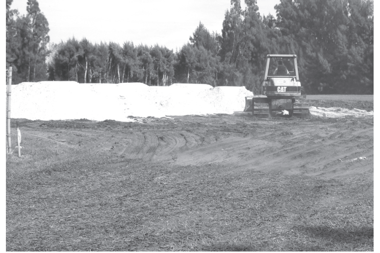
Bulldozer grades the foundation.
