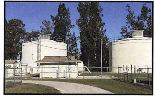
Primary Water Plant
