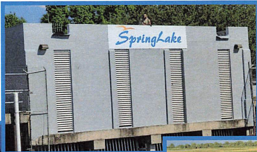
Pump station gets painted and a new sign installed
