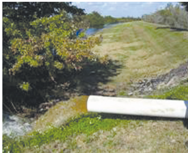
Water was drained from the existing canal.
