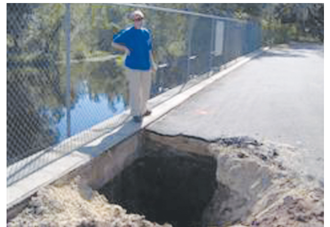
Angela Hendrichsen with SFWMD inspects the sinkhole.
