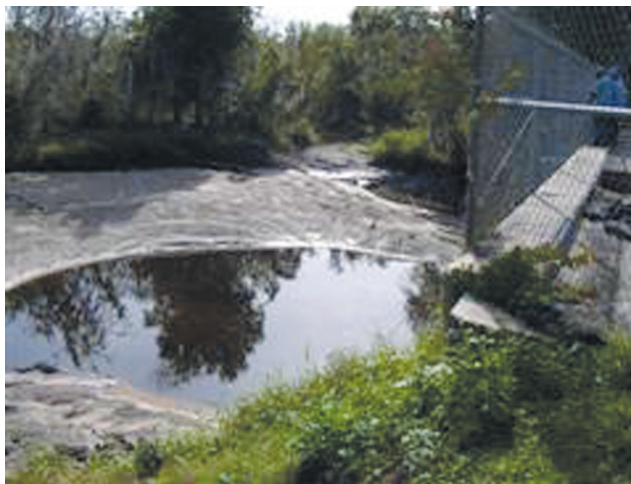
The channel was drained to able a physical inspection of the pump.
